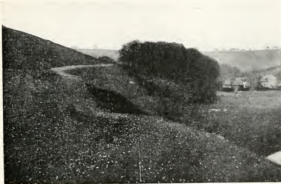
XX.—VIEW OF THE SAME ROADWAY BUT LOOKING IN THE OPPOSITE DIRECTION.
